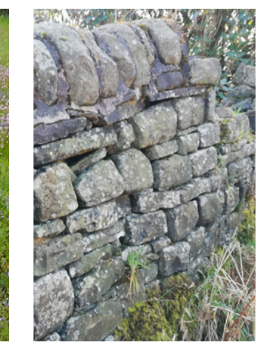
Retain existing drystone walling where feasible
